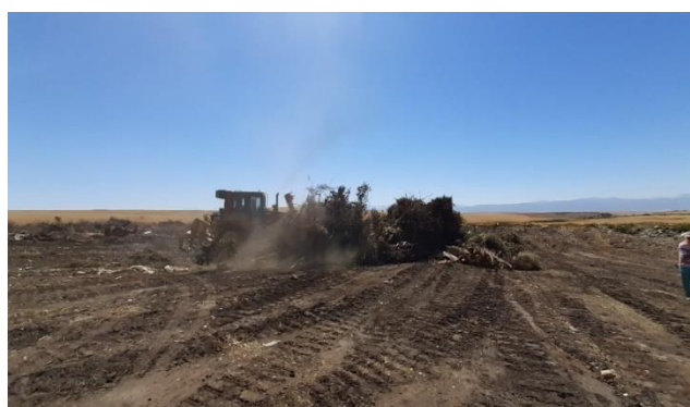
Photo of landfill site being cleared.
