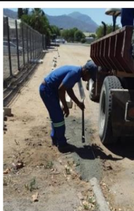
New road construction
