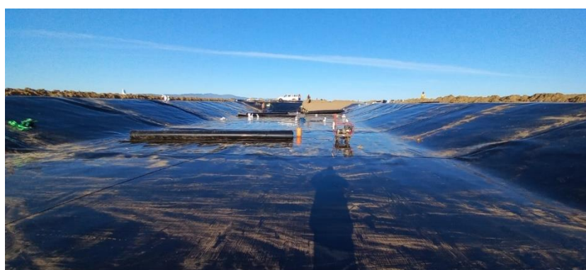
Upgrading of Dwarskersbos Sewerage Works
