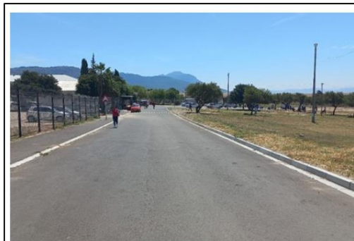
Bitumen road construction
