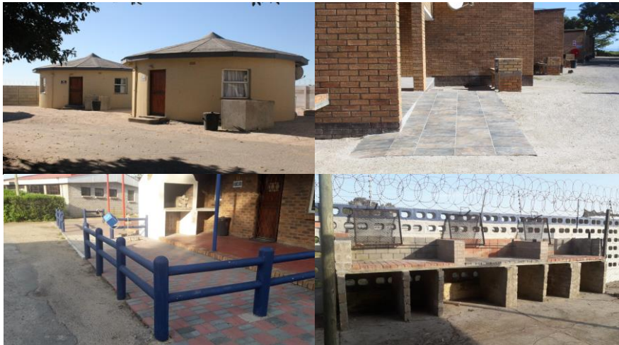
Regular Maintenance at Holiday Resorts
