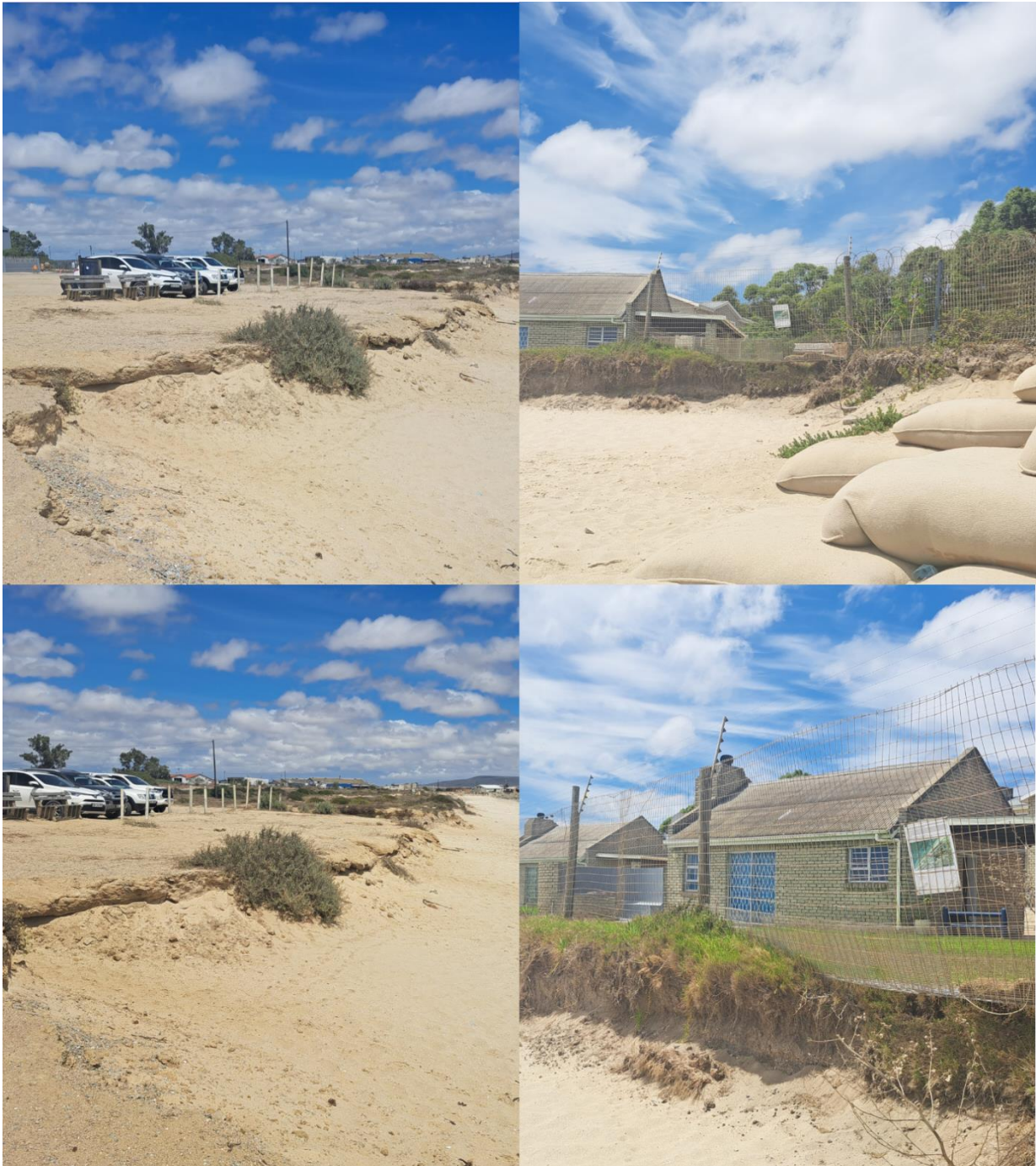
Figure 40: Coastal erosion in Laaiplek.
