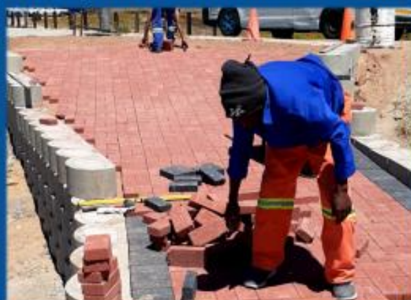
The Walkway RSEP project in Velddrif was completed in March 2021
