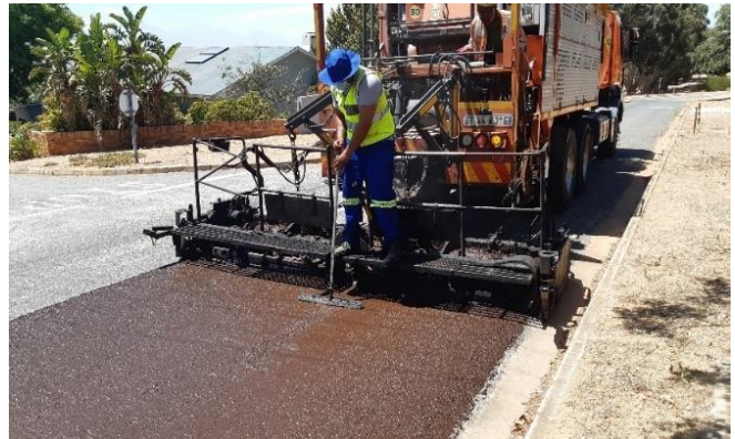
Road being resealed in Piketberg as part of preventative maintenance
