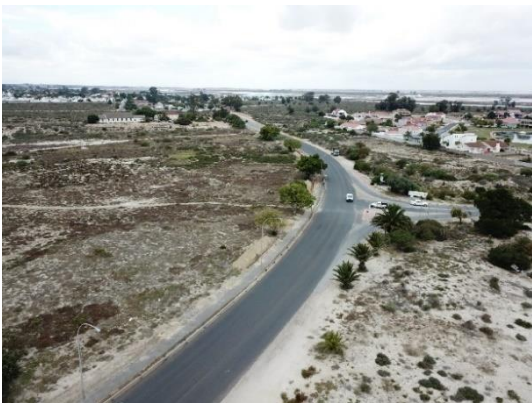
Section of Voortrekker Street in Velddrif resealed
