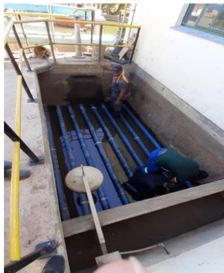
Piketberg WTW filter media being replaced
