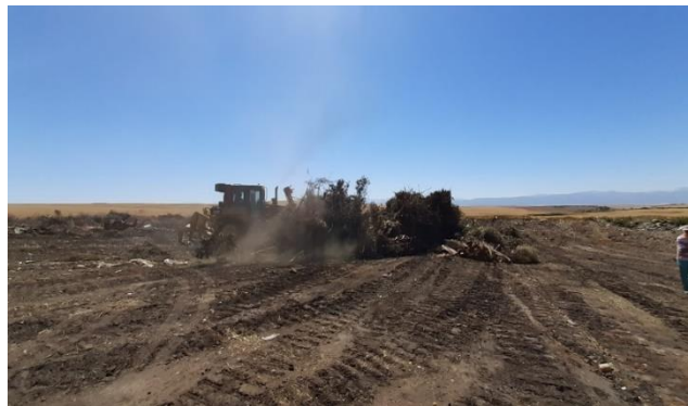
Photo of landfill site being cleared
