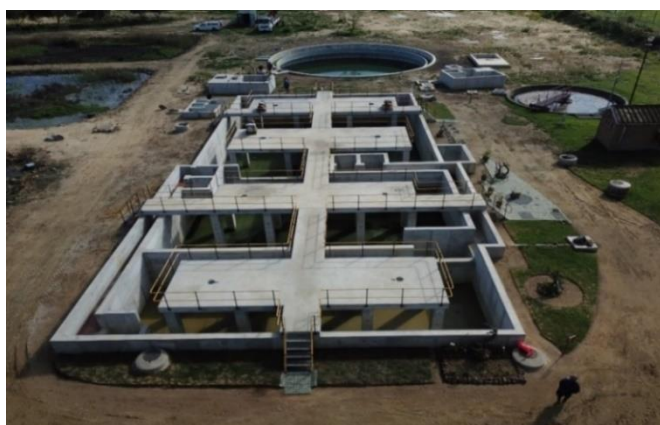
Upgrading of Porterville Sewerage Works
