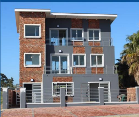
The Active Box in Piketberg valued at R2,6 million completed in 2020
