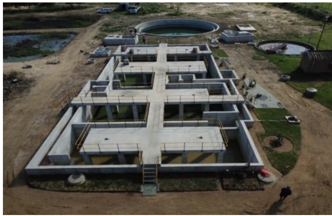
Upgrading of Porterville Sewerage Works
