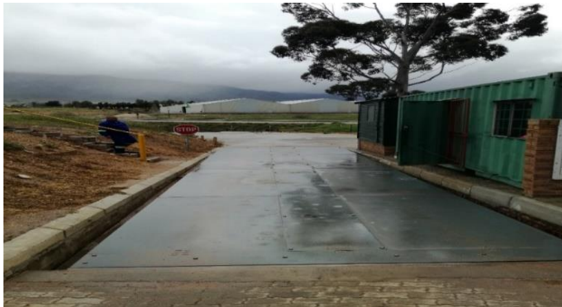
Photo of weighbridge
