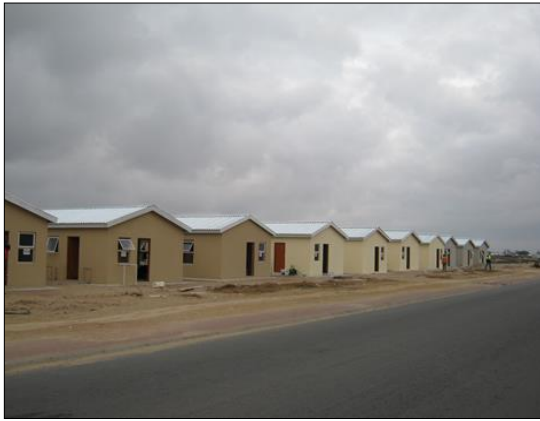
Construction of 30 houses in Velddrif
