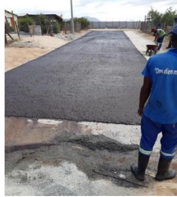
Upgrade of gravel road - Aurora
