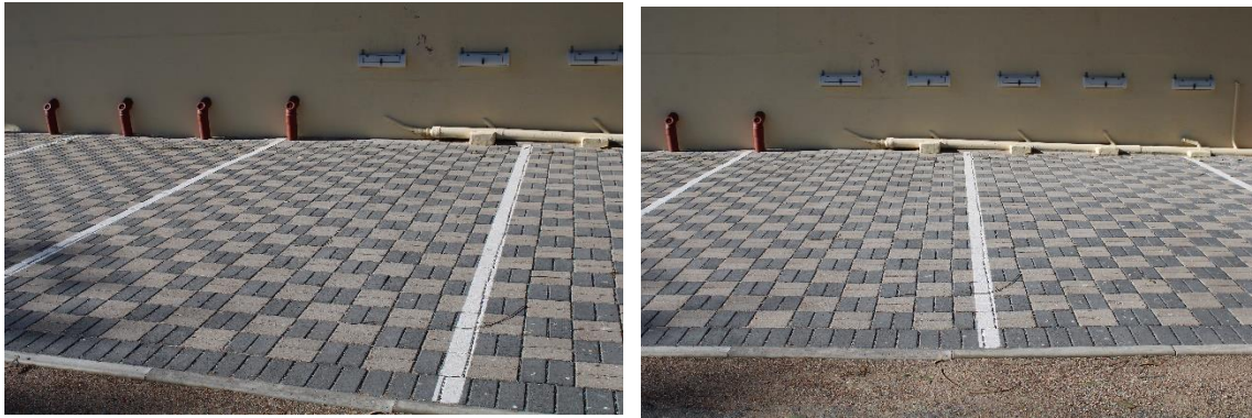
Paving at Stywelyne beach resort
