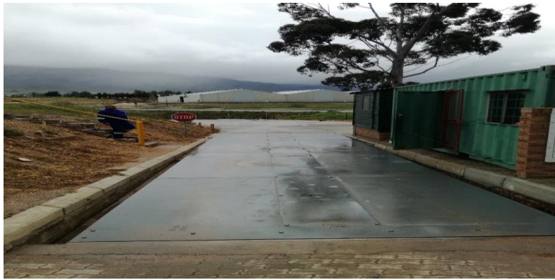
Photo of Weigh Bridge
