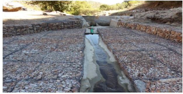
Inlet works Wittewater and rock paved canal
