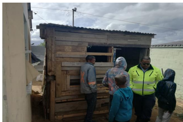
Law Enforcement busy with the removal of illegal structures
