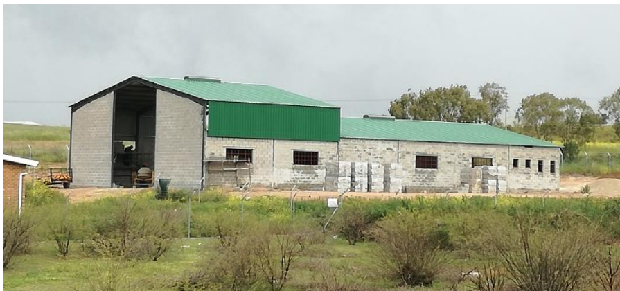
Photo of recycling plant under construction: Piketberg
